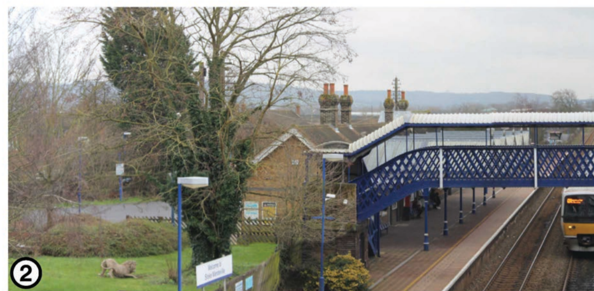
2 A4010 Station Road bridge looking south-east towards the Site
