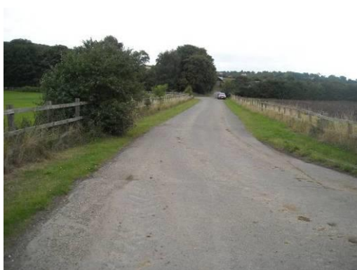
Fig. 12 Metalled access road
