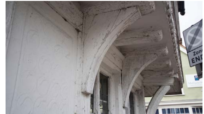
Photo 30: Ornate jetty on street-facing building
