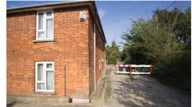
Photo 1: View of lane facing towards Radwinter road on east side
