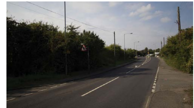
Photo 3: View looking west along Radwinter road from site entry
