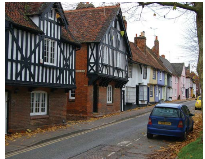
Photo 39: Former almshouse on Castle street, Saffron Walden
