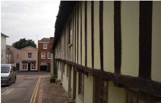
Photo 49: Tudor houses opposite the church
