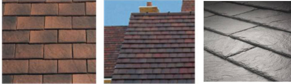
Roof materials are a mixture of reconstructed slate and plain tiles
