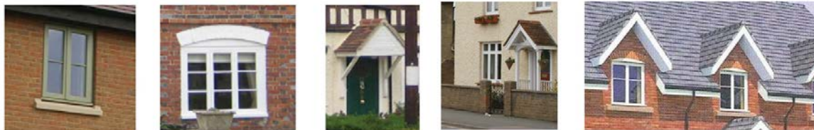
Casement windows with cottage style arched brick headers and pop-up dormers
