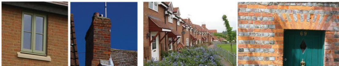
Cottage-style windows, roof styles and details
