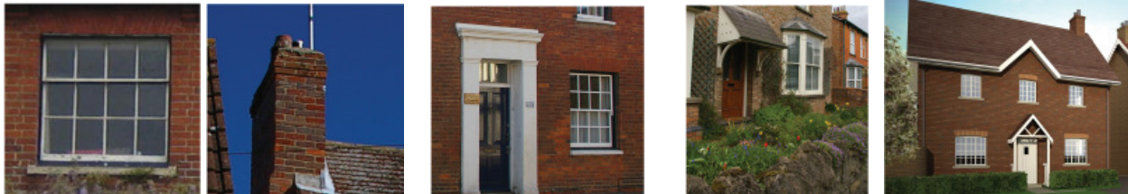
Semi-formal details: Less elaborate than the boulevard character but more elaborate than the green edge character
