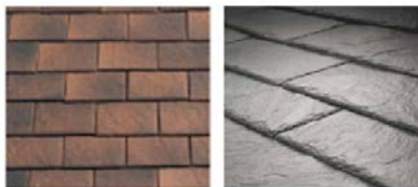
Roof materials are a mixture of reconstructed slate and plain tiles
