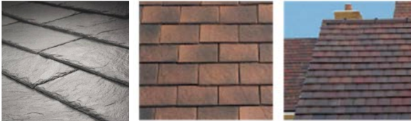
Roof materials are a mixture of reconstructed slate and plain tiles
