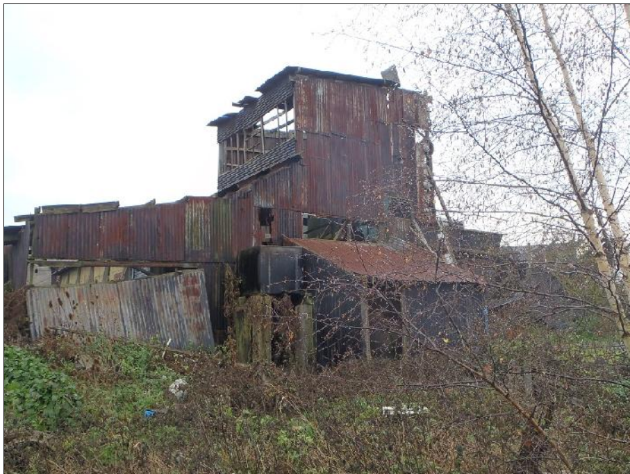
The derelict building adjacent to the south-eastern corner of Field C.
