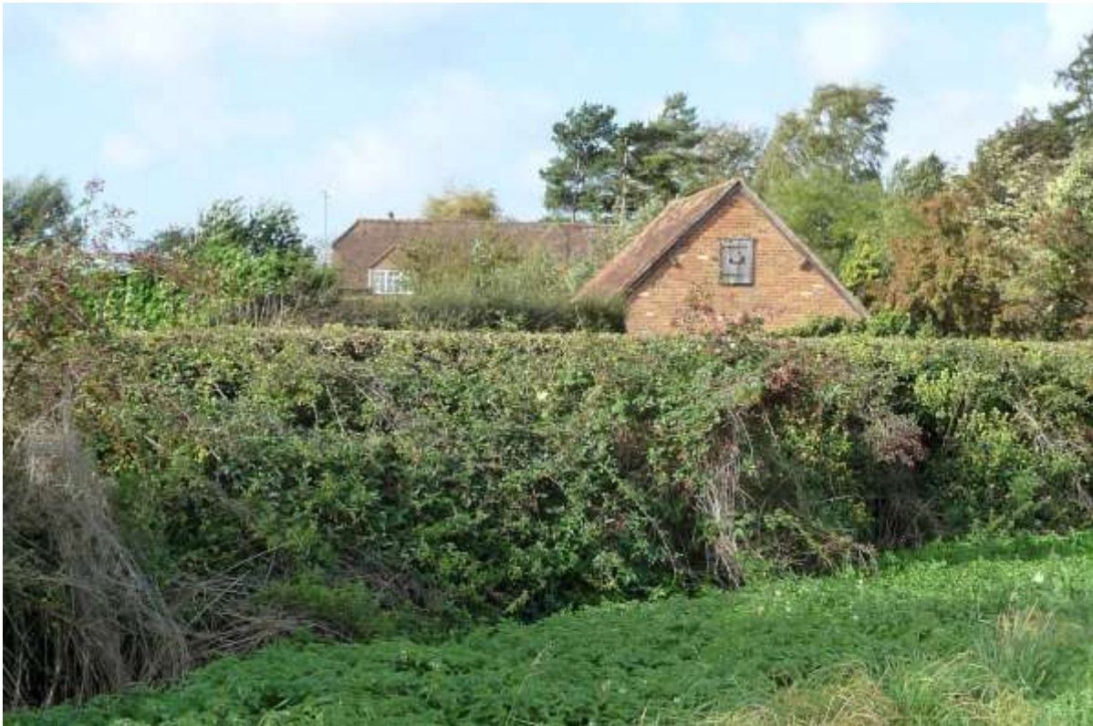
Plate 23: The limited view of the roof of the heavily converted Willow Barn behind its garage/outbuilding as seen from close to the south-west boundary of the site
